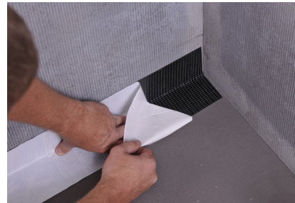
Image 2: Floor to wall edge seam
