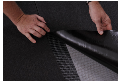
Image 1: Floor Installation butt-joint membrane seams
