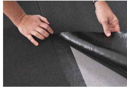
Image 1: Floor Installation butt-joint membrane seams
