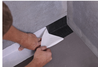
Image 2: Floor to wall edge seam
