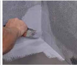
Apply SubSeal® over PF corner
