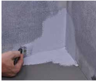
Apply SubSeal® to corner
