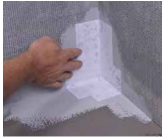
Place PF Corner into position
